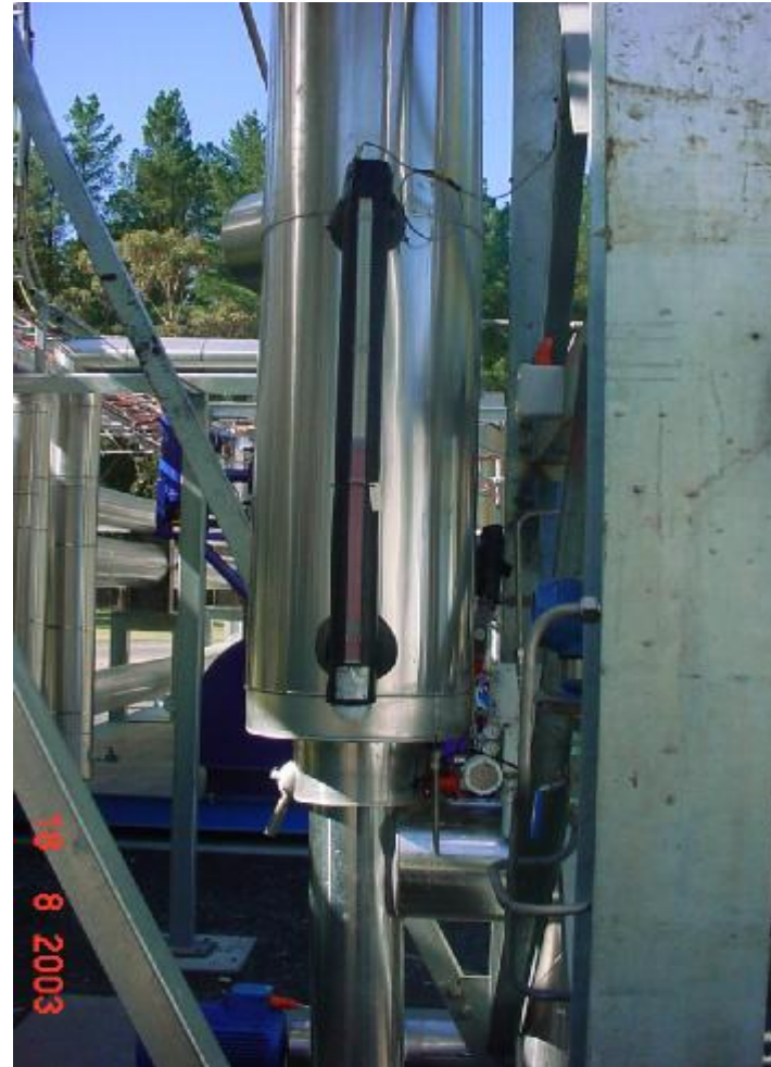
Models with insulation for application with media below zero
