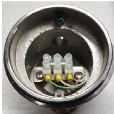
Typical internals of wired large 240V junction box
